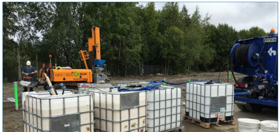
Fig. 5 and 6 - Injection works on site
