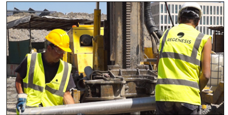
Fig. 5, Drilling wells prior to injection in Area 2
