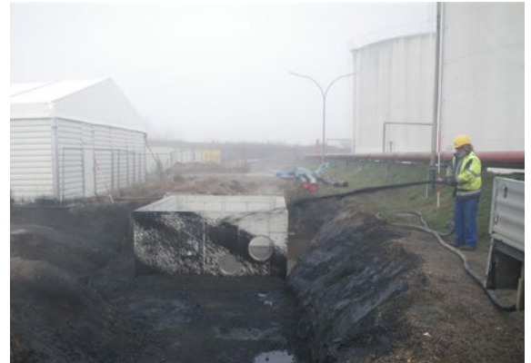
Fig. 5: PetroFix spray application
