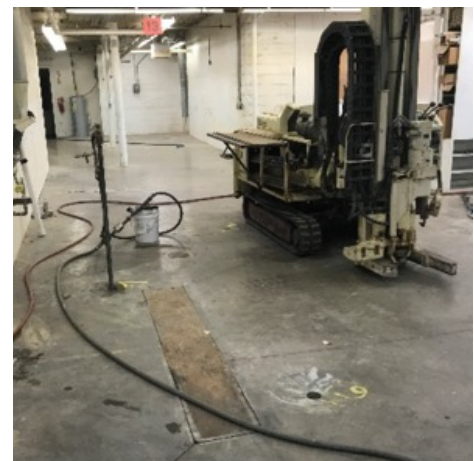
PlumeStop Injected at Multiple Points Simultaneously
