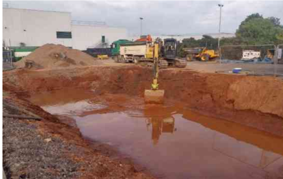
Fig. 2 Excavation in the source area (by others) © Golder
