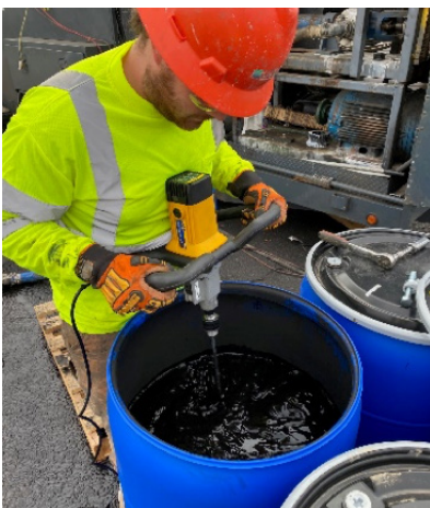
Homogenization of PetroFix using a hand-held paddle mixer
