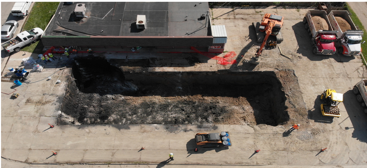
Example of a PetroFix application in an excavation
